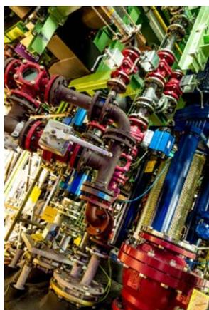
Supply lines for a 12 cubic meter reactor in the central organic pilot plant of Saltigo GmbH in Leverkusen. Photo: Saltigo GmbH
