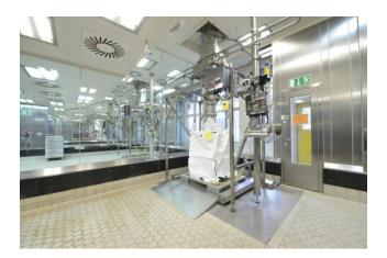
Solids filling of intermediates and active ingredients in big bags at Saltigo GmbH in Leverkusen under cleanroom conditions. Photo: Saltigo GmbH
