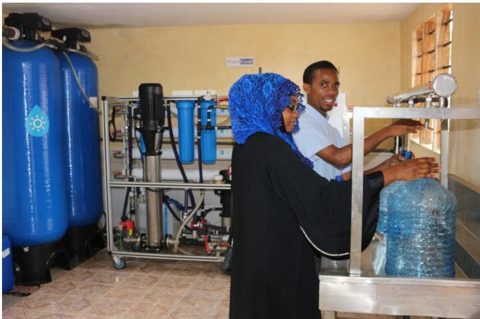
Solar-powered reverse osmosis membrane elements from LANXESS' Lewabrane brand are used in the village Burani; Kenya, to turn raw water with a high salt content of 4,800 ppm into potable water.
