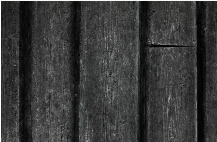
The concrete, which is colored with black iron oxide pigments of LANXESS' proven Bayferrox brand, reproduces the weathered material wood.
