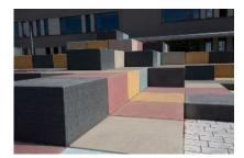
The concrete cubes that make up the "Urban Star" are designed with a flat, pyramid-shaped pitch on their surface, which prevents water from accumulating and minimizes the risk of ice forming in the winter.
