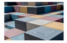
The translucent-concrete cubes are crowned with a horizontal slab that is made from smoothed, anthracite-colored standard concrete and can be easily accessed for inspection purposes. Photo: LANXESS AG
