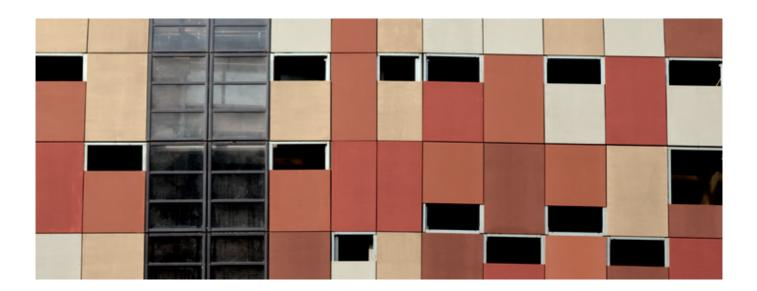
■ The unique façade was created using panels of through-coloured glass-fiber-reinforced concrete.
